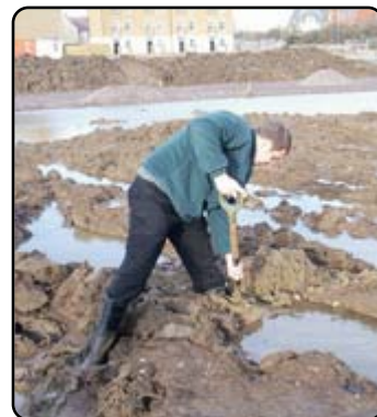
A Landscape Contract Manager trying to release water in footings for a path!
