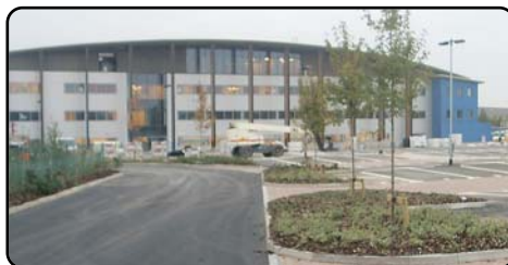
Gloucester FM Services, Quedgeley
